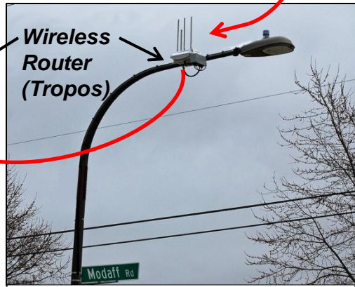
Streetlight with wireless router
