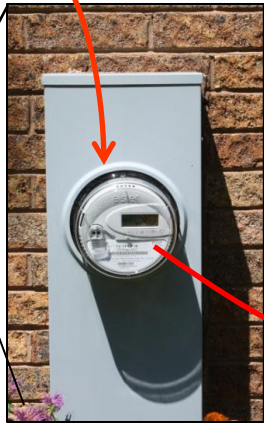
Smart Meter sends signal
